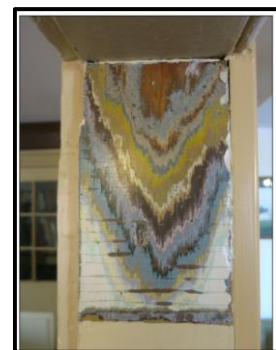
Paint layers on a door jamb.
