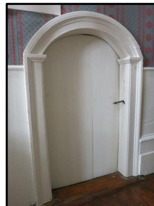
Smoke Chamber Door
